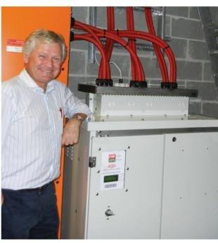
Wilson's 750 kVA Voltage Power Optimiser installed in Melbourne
